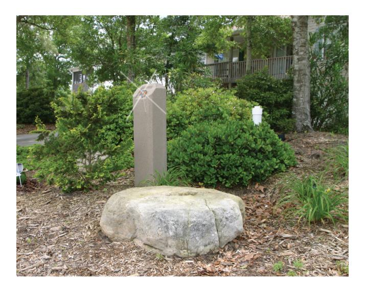
The solar light monitor is easily visible from a long distance, avoiding the need for operators to physically check every vacuum valve in the system.
