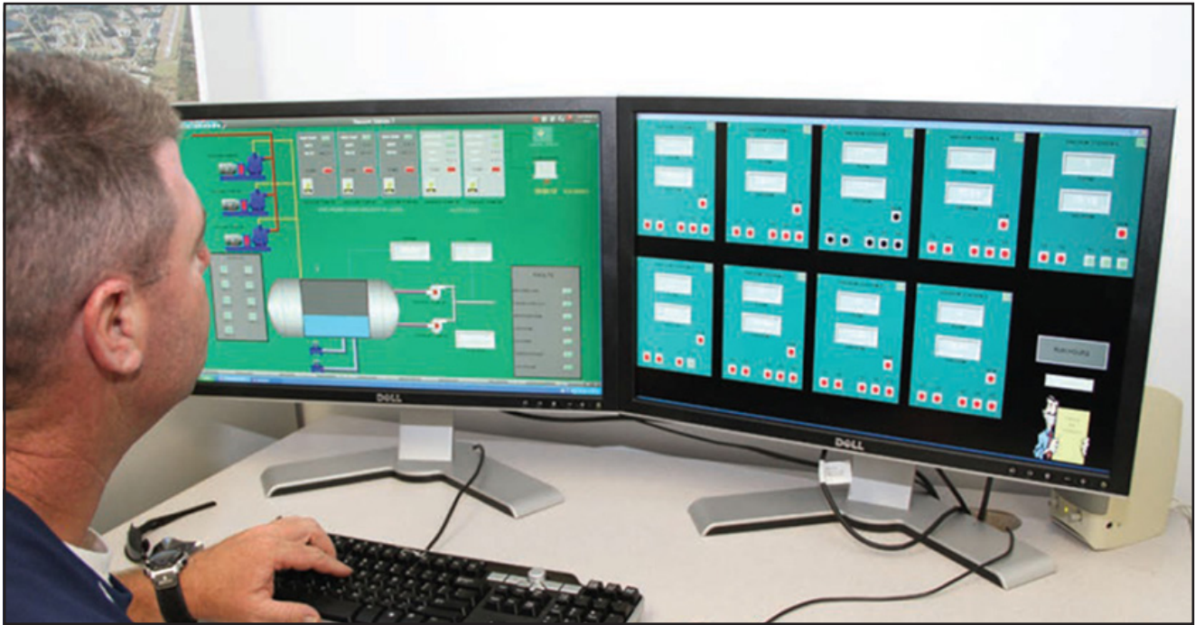
CONTROL CENTER – One person can control most aspects of Oak Island’s vacuum sewer system from a central command center. Here, the operator can see the status of each of the city’s nine vacuum stations and make adjustments to any one of them.
