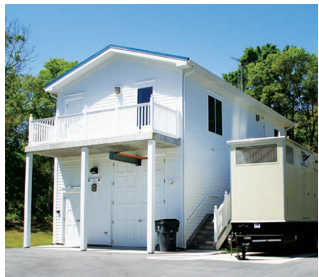
VACUUM STATION – This is one of Oak Island’s nine vacuum sewer stations. In the event of a power outage, the stations can be powered by a portable generator.
